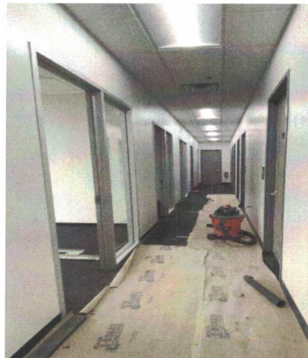
Inside office Single wooden door with side light glass pane on side. Please refer to floor plan for door swing and side light orientation. (framing needs to be same as the front double door)
